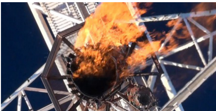
Flare tip inspections
